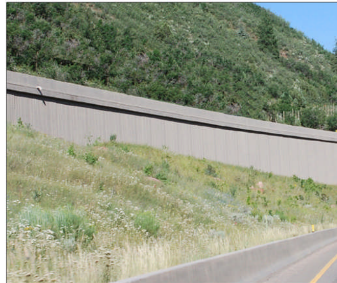
C | Incorporate earthwork solutions in conjunction with structured retaining to limit the height of retaining walls.
