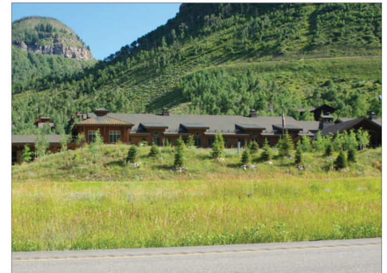
C | Where possible, earthwork and landscaping should be utilized to buffer community-based land uses from the corridor rather than stand-alone sound walls.
