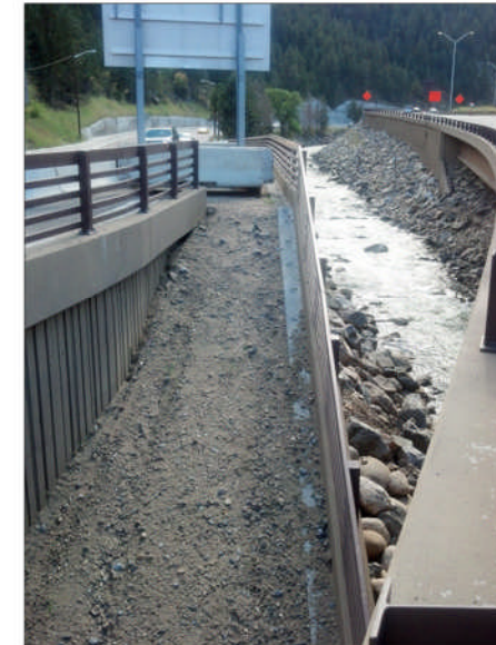
D | A wildlife ramp adjacent to Clear Creek at I-70 and Central City Parkway allows safe access for animals under I-70.
