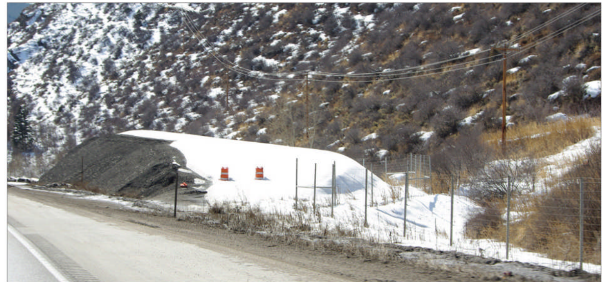
B | Construction and maintenance materials should not be stockpiled along medians or shoulders. This is especially important for areas with high visual or recreational value.
