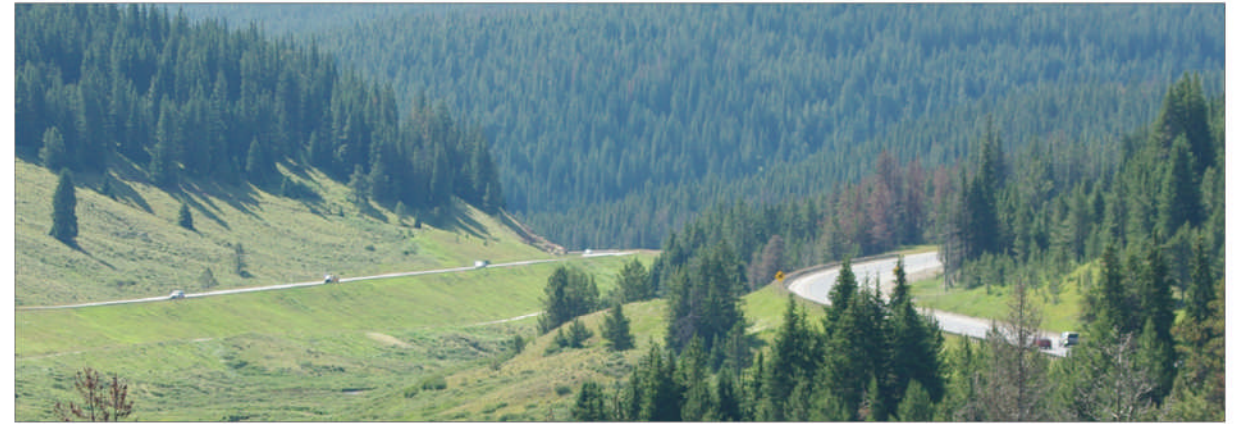
A | Medians of variable width blend the transportation corridor with natural landscape and drainage patterns.
