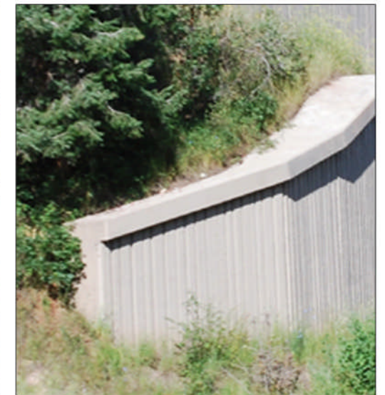
D | Turning the ends of walls helps integrate them into the adjoining slope.
