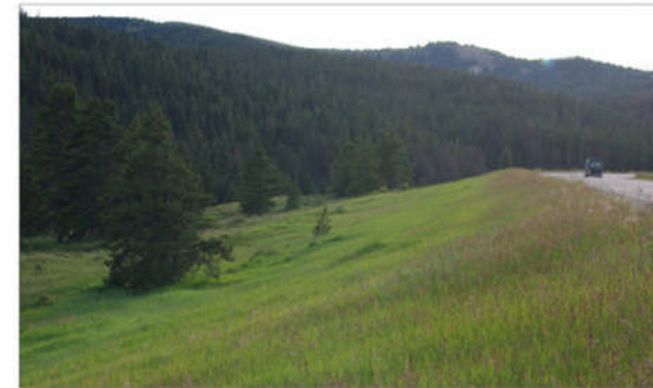
A | Rounding the top and toe of the slope blends embankments into the existing landscape and facilitates
