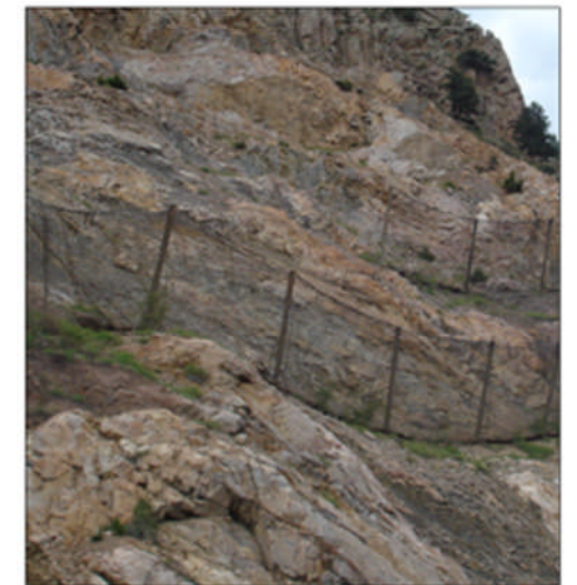
D | Rock fall protection devices, when required, follow existing contours and reduce visual clutter.
