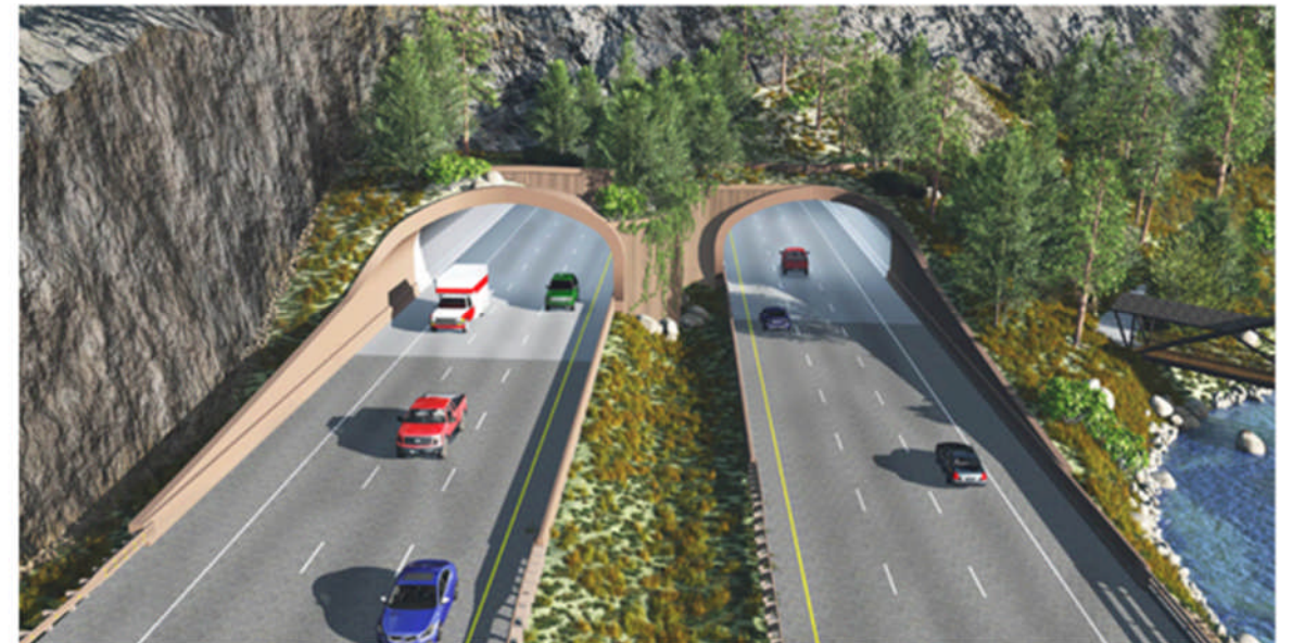
C | The transportation facility at the Twin Tunnels aids in rock fall protection by incorporating rock fall protection into design of retaining walls, noise wall, grading and landscaping.
